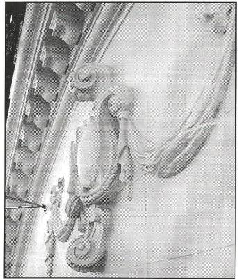
had been badly eroded. Metropolitan called upon a local sculpture/artisan to craft positive reproductions of some of the deteriorated architectural pieces and in turn created molds in-house in which to cast the new elements.
