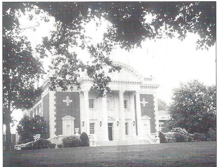
Worcester Academy's historic Warner Theatre was recently restored, in accordance with sound waterproofing techniques.
