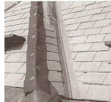
A new slate roof was installed with newly fabricated copper valleys
