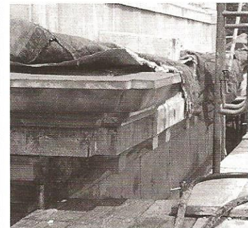
Complex formwork (e.g. outside cornice with inside corner)
