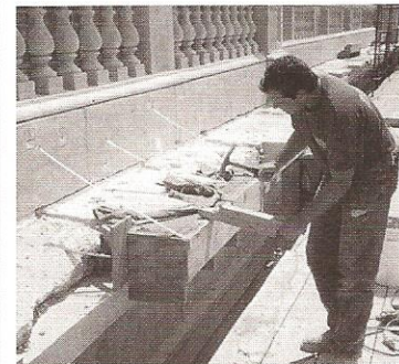
Cast cornice work – upper perimeter at parapet wall
